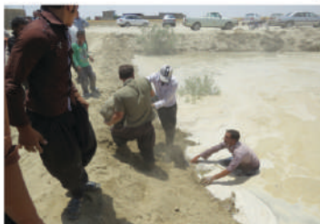
RIVER DREDGING NEAR WETLAND
